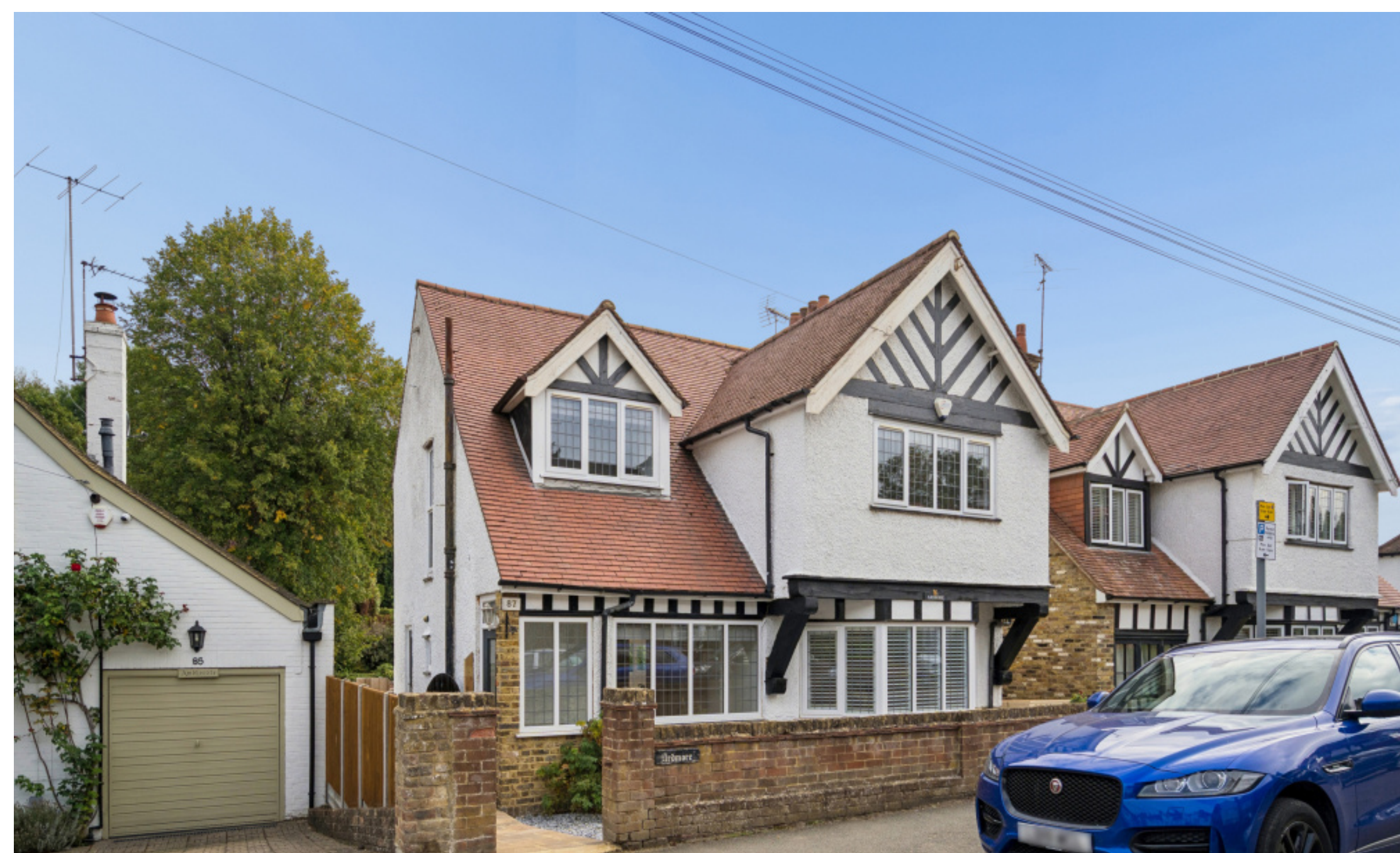
A refurbished four bedroom home in the heart of Chorleywood village Lower Road, Chorleywood, Hertfordshire WD3 5LA
